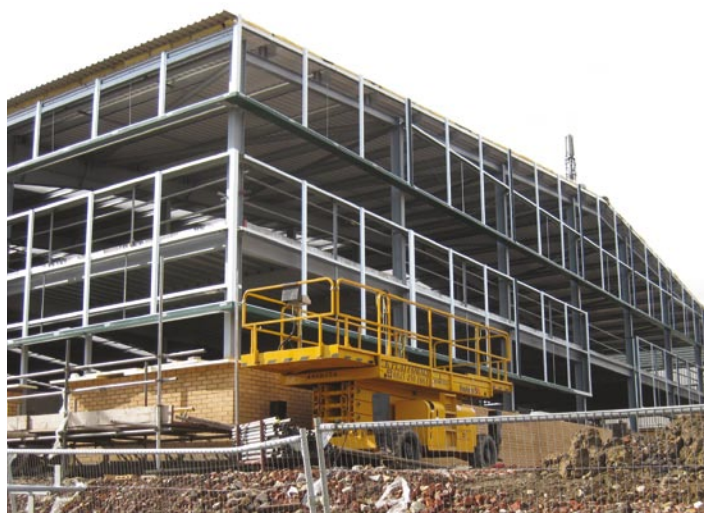
New Metflex factory being constructed. Completion date: September 2010.
